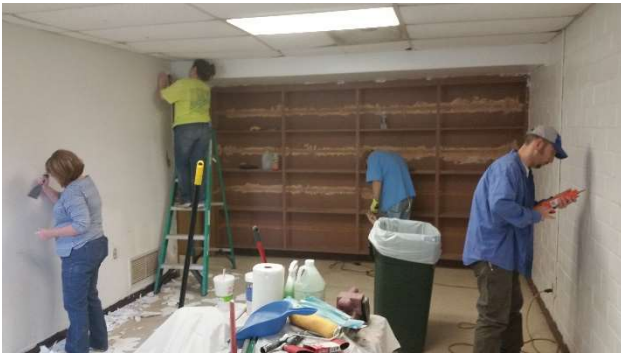
Old Armory Comm Room in work. Good job folks!
